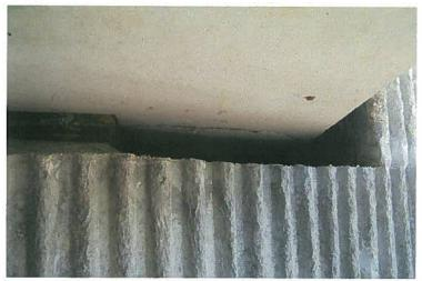
Photo 15 - NW bearing and delamination at bottom of girder
