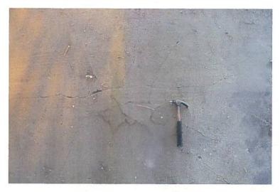
Photo 31 - under-bridge sidewalk delamination
