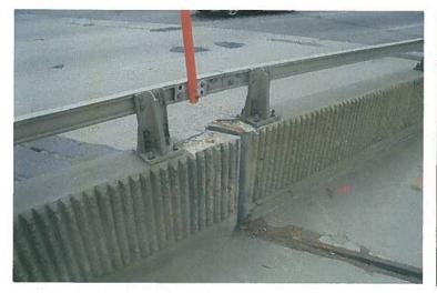
Photo 13 - north traffic back wall at west expansion joint
