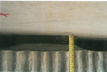
Photo 14 - NW bearing and delamination at bottom of girder
