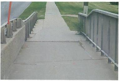
Photo 9 - south sidewalk east end trip hazard
