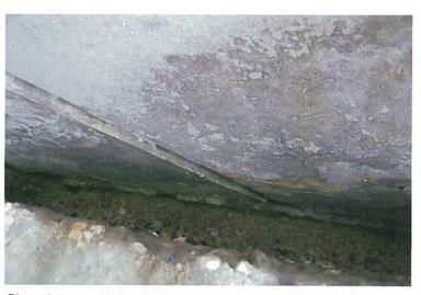
Photo 2 - west abutment gravelly material on seat
